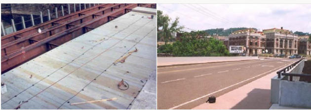
Figure 2: Market Street Bridge (Wheeling, WV, built in 2000) with FRP decks (WVU).
