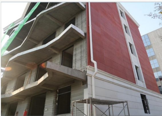
Figure 4: 6-story 3D printed apartment building (Sevenson, 2015).
