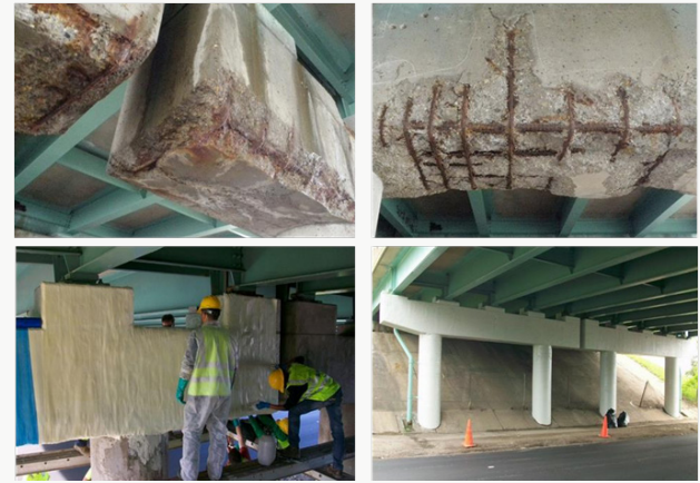
Figure 3: Rehabilitation using FRP wraps of Madison Avenue Bridge, Huntington, WV (WVU, 2014).
